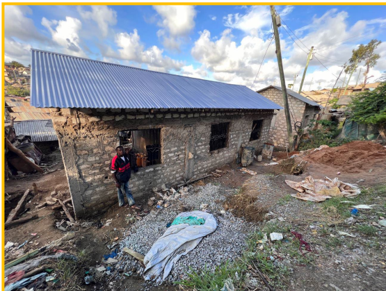
The boys’ new house with a new roof
